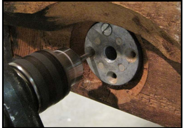
New socket being installed.
